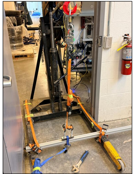
(Tensile Experiment Setup) Electrical support systems visible in background
